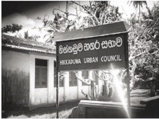
Figure 1 - The flood-damaged library shortly after the Boxing Day tsunami 2004
